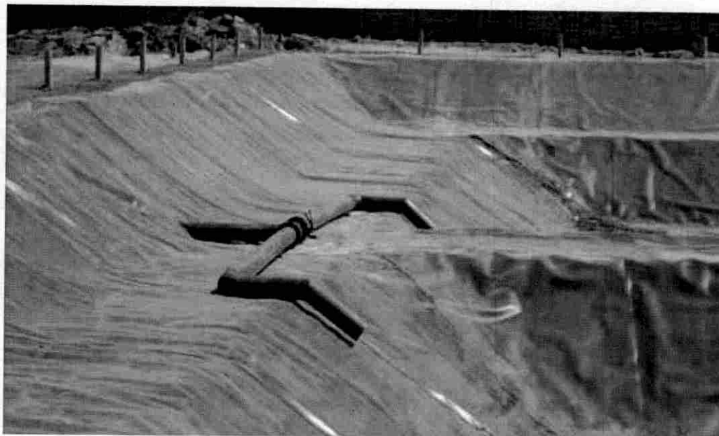
Figure 4.10: Sealed Leachate Pond with Two Basins 14
