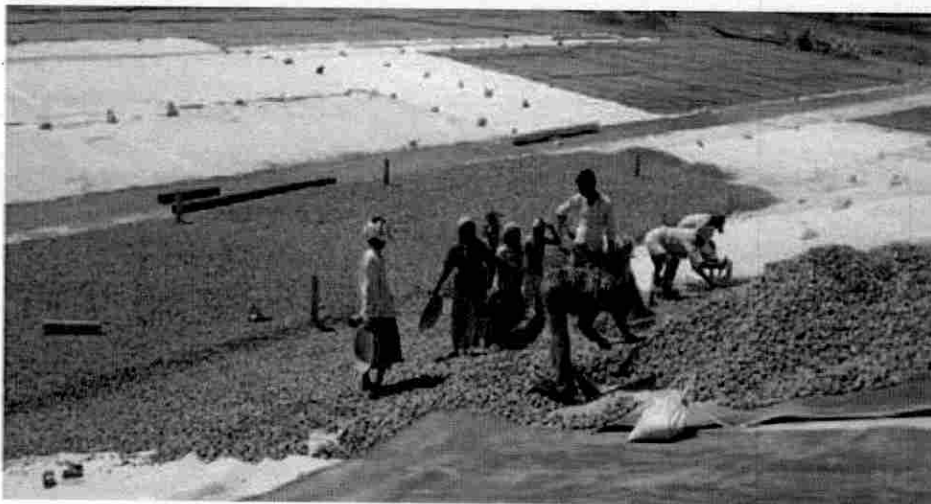
Figure 4.13: Sanitary Landfill under Construction 17
